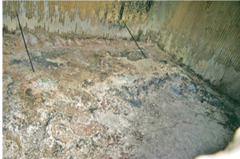
Figure 4. Bed after shutdown with thermocouples installed
