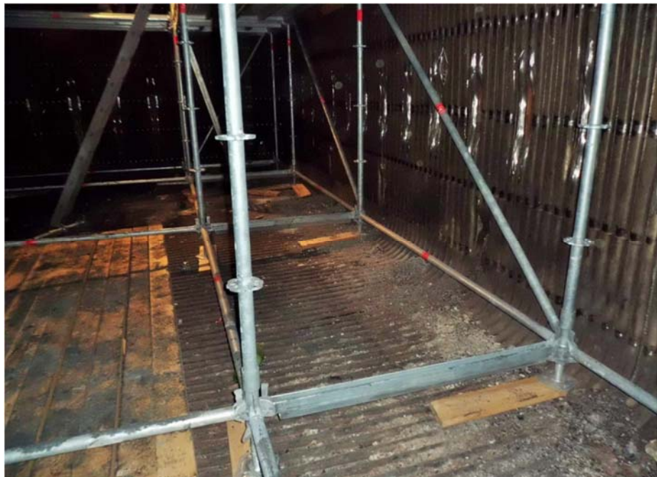
Figure 8. Floor after washing in a recovery boiler with 3600 tDS/day capacity
