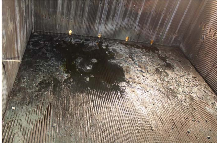
Figure 7. Floor after washing in a recovery boiler with 1600 tDS/day capacity
